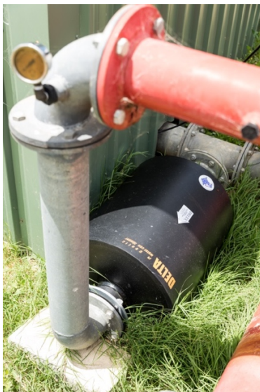
A magnetic water conditioner applied just downstream of a pump.
